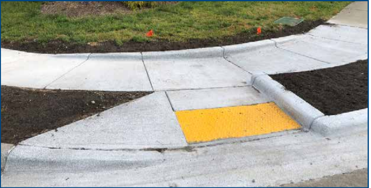
PROWAG Compliant Curb Ramp Example Source: City of Durham
